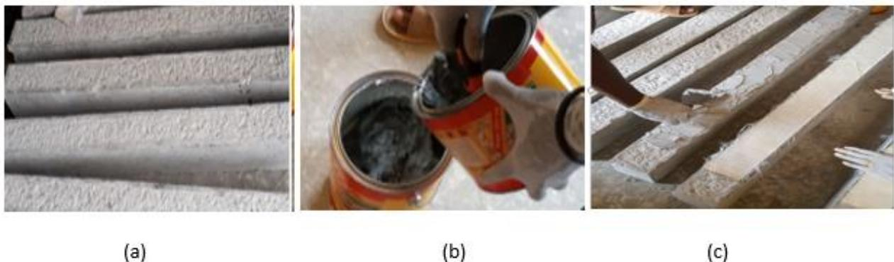
Fig. 1. Strengthening Process: (a) Roughing the Surfaces of the Beams (b) Mixing Adhesive Substance (c) Bonding of GFF to the tensile surface of the beam
