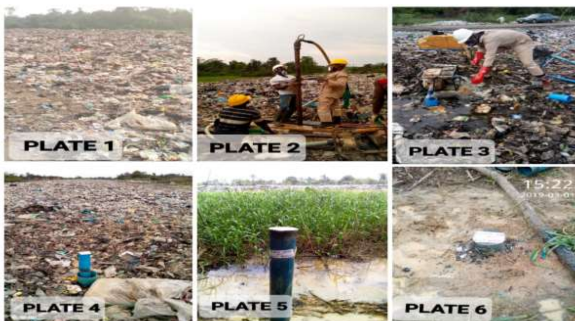
Figure 1.0: An Array of Activities within the Dumpsite Showing Active Drilling and some Drilled Boreholes
